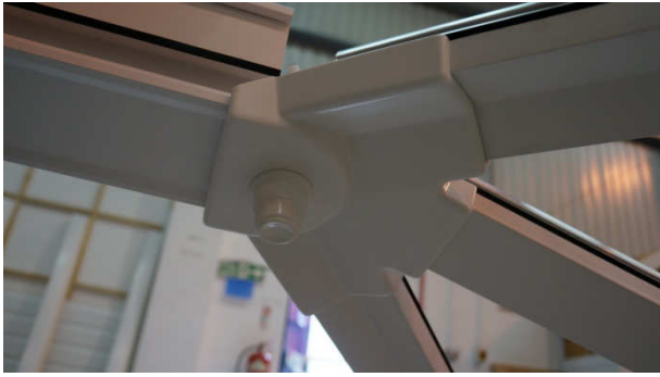
12. Position the spider bottom cap and fix using decorative boss onto nylon threaded bar.
