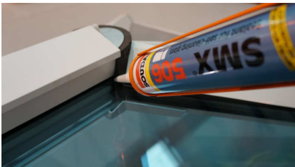
16. Fit the rafter and hip top caps using a nylon mallet and seal around perimeter of foam bung. ONLY use compatible sealant with self cleaning glass, Soudal SMX 506 is recommended and available from Eurocell Branches.
